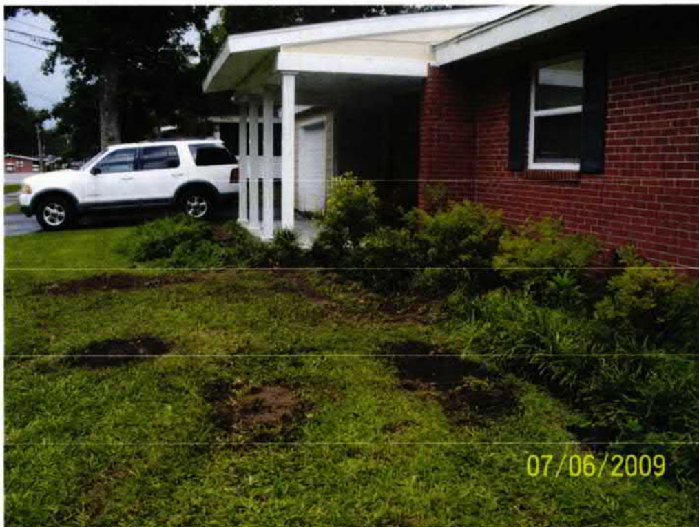
Picture 2: Site after completion of work.
